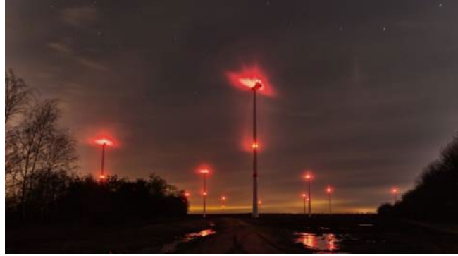
Fig. 2: Horizontal axis wind turbines require massive installation infrastructure, require flashing lights for towers over 200
