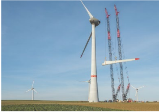
Fig. 2: Horizontal axis wind turbines require massive installation infrastructure, require flashing lights for towers over 200
